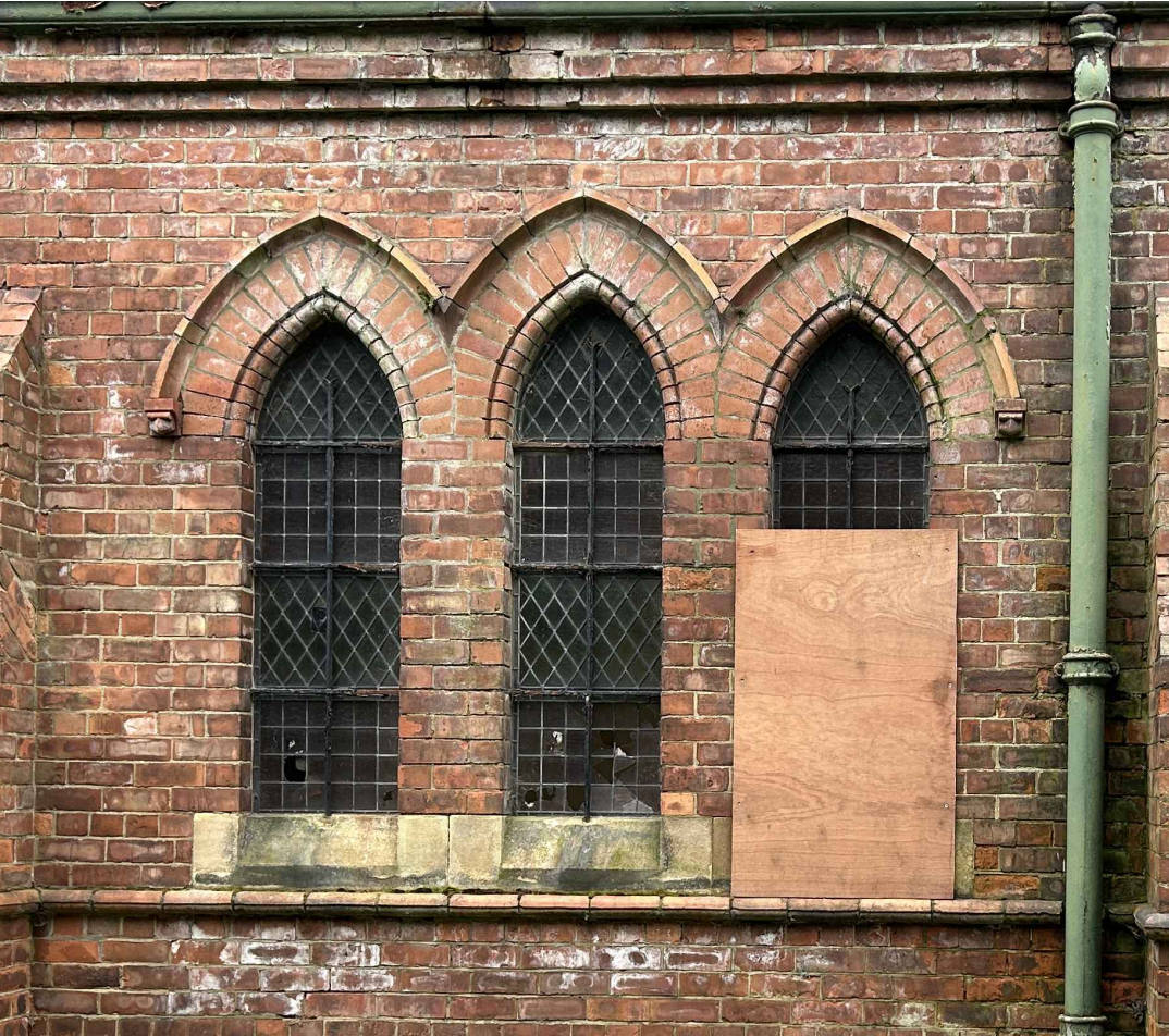
Typical existing window condition - the building has suffered from vandalism over the last few years since it has been vacant and many windows now require substantial repair/ restoration works.
