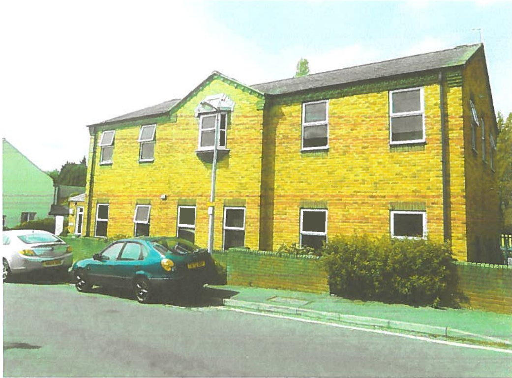
Photo 6 – Existing commercial property at 14 Leonard Street
