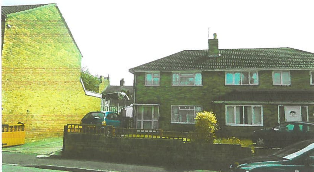
Photo 4 – Existing properties 19 & 21 Leonard Street
